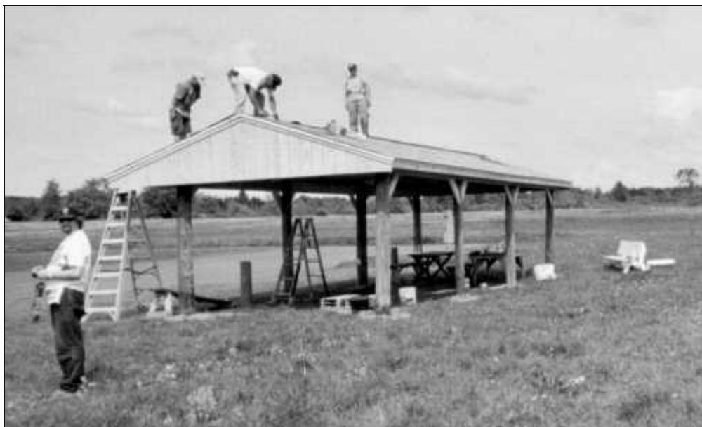
Adding the finishing touches
