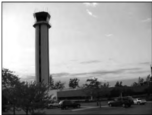
160 foot observation tower
